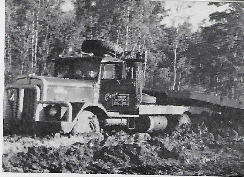
Most powerful diesels could not move through mud
